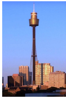
Fig.9 AMP Tower Sydney, Australia
