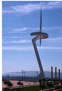
Fig.10 Montjuïc Communica- tions Tower, Spain
