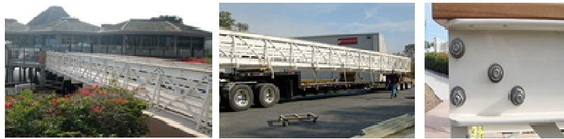
Fig. 1. Fully assembled 20m bridge
