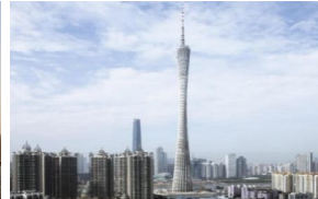
Fig.7 Canton Tower, Guangzhou
