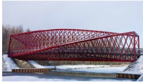
Fig.3. Horizontal "twisted" bridge in Netherlands
