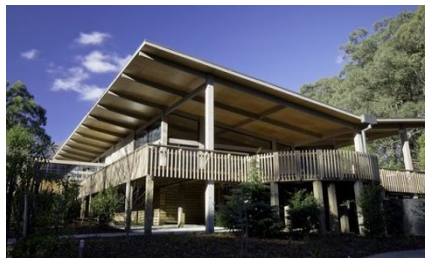
Fig.3 Smith and Tracey Architects' Olinda "Tea House" in Melbourne
