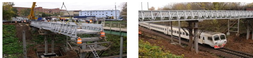
Fig. 2. Fiberglass bridge near the railway station Chertanovo, Moscow
