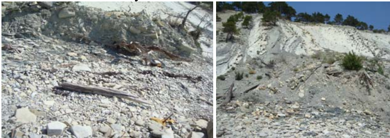
Picture 2: Landslide at point 11 in 2014
