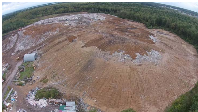
Fig. 2 The landfill “Kulakovo” condition (the data as of 29.09.16) [2]
