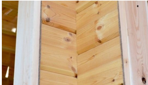
Fig.1 Glued laminated timber wall
