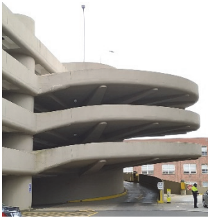
Figure 7. The ramp fence in the form of a helical strip
