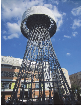
Figure 11. One of the few lattice water towers of V.G. Shukhov in our days, Krasnodar, Russia
