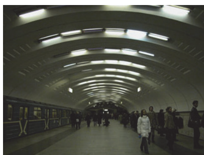
Figure 4. Babushkinskaya metro station, Moscow, Russia, 1978. The illumination of the station is provided by lamps, which are located in the slots of the elliptical arch
