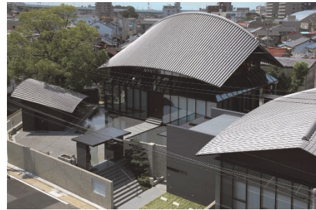
Figure 14. Different types of roofs from corrugated metal in the form of cylindroids, "Ishibashi, Tokugawa & Associates", Tokyo, Japan
