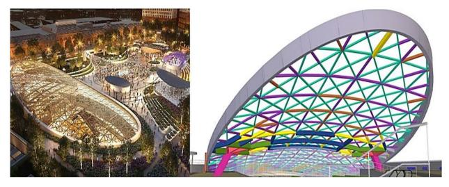
Figure 7. The shape of a large dome in the shopping center "Paveletskaya Plaza"
