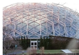
Fig. 3. St. Louis, USA. Geodesic dome "Klimatron", used as a greenhouse of the botanical garden (height 21 m, diameter 53 m). Made in aluminum structures. 1960
